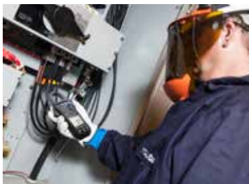
Analyze Power-related Issues
